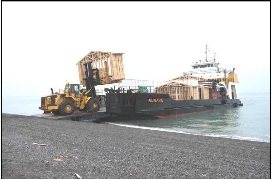
A framing package is unloaded from the Nunang as it waits in the port of Brevig Mission.
